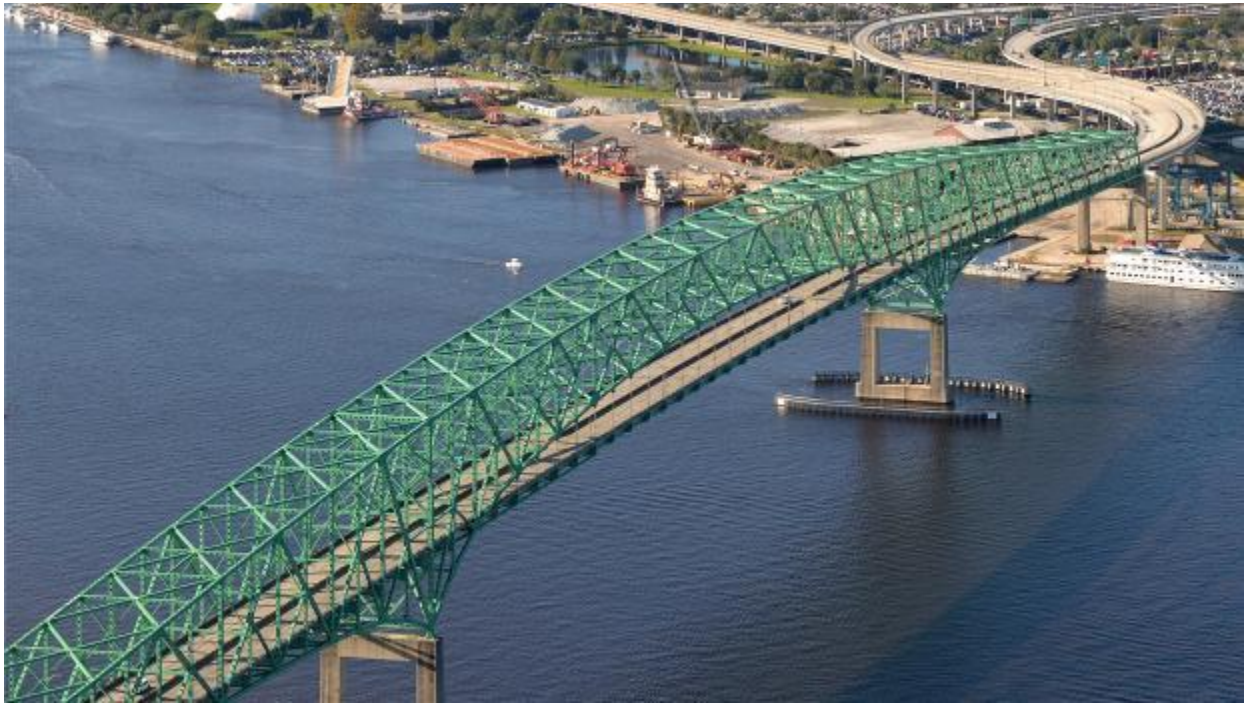
Hart Bridge, Jacksonville, Florida
