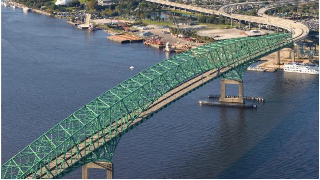
Hart Bridge, Jacksonville, Florida
