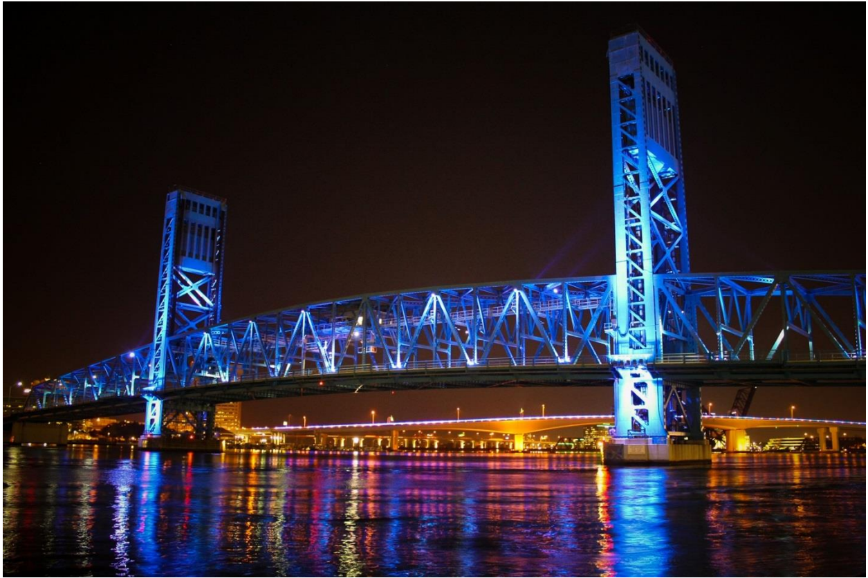
Main Street Bridge, Jacksonville, Florida
