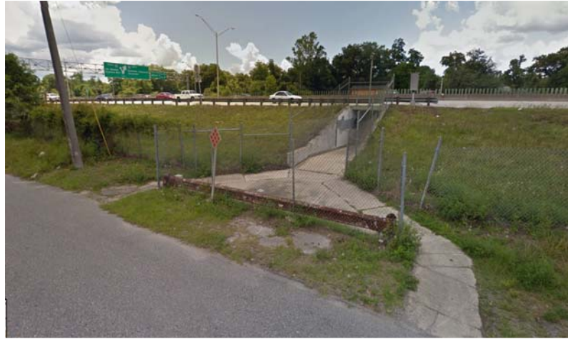
Day Avenue pedestrian underpass. View looking south from Waller Street.
